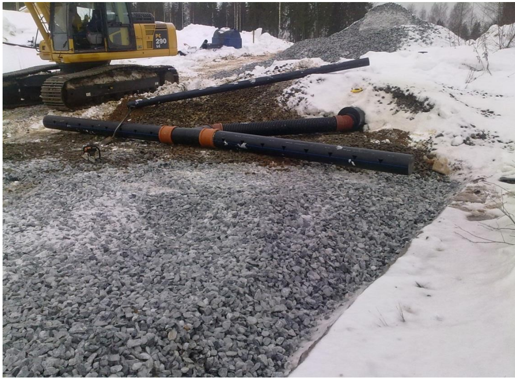
Photo 6 Installation of the water distribution pipe to the treatment plant photo Timo Järvinen 2010
