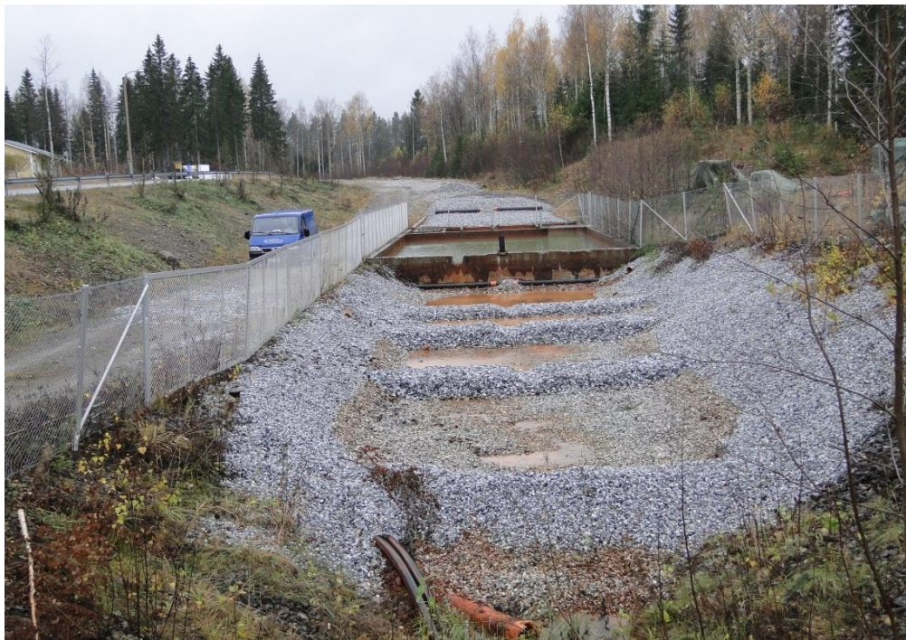
Figure 7 Kotalahti mine wastewater treatment plant. Closest to the wet filter, the former sedimentation basin. photo.Timo Järvinen 2010
