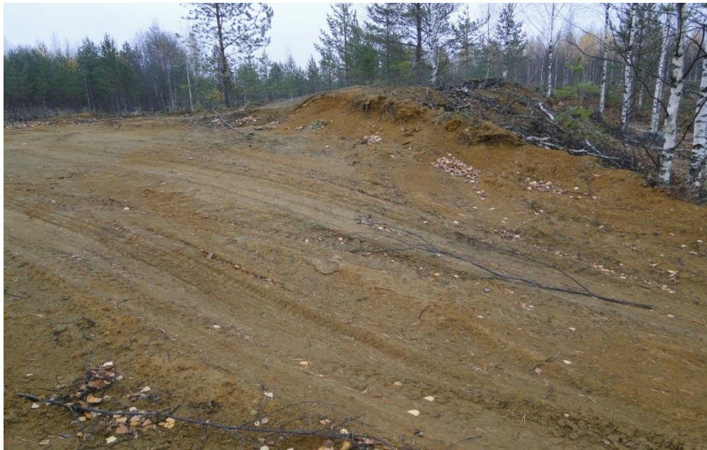
Figure 8. The tailings dam before the application of the sewage sludge.
