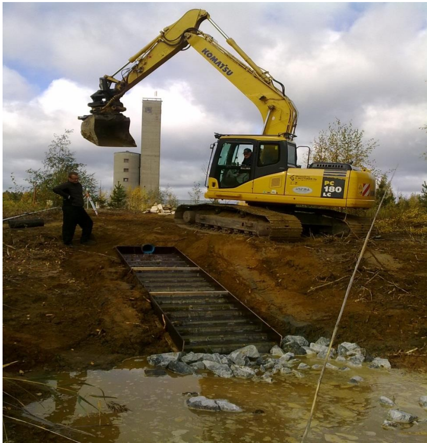
Figure 15. Installation of the test pumping discharge pipe and the wooden aeration drill in Basin C. Photo. Timo Järvinen 2009
