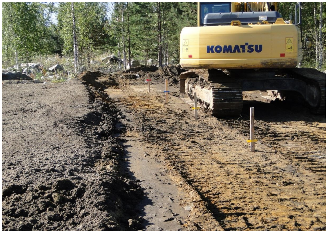
Figure 12. The left side of the picture shows the filled test area number 1. and the machine fills test area number 2. The piles are marked with layer thicknesses of 20-, 30-, 40- and 50 cm. Photo by Timo Järvinen, 2010
